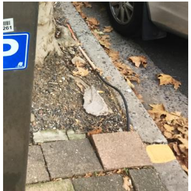
Figure 6: black cable housed in orange conduit
