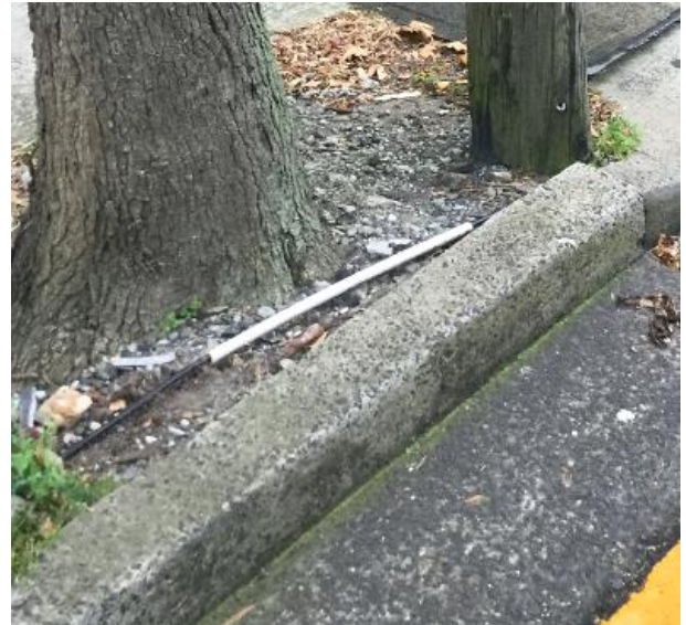
Figure 4: black cable housed in white conduit
