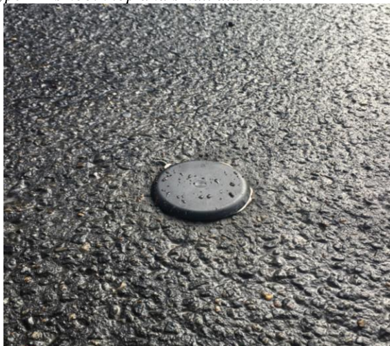
Type 2 – smooth top and small diameter
